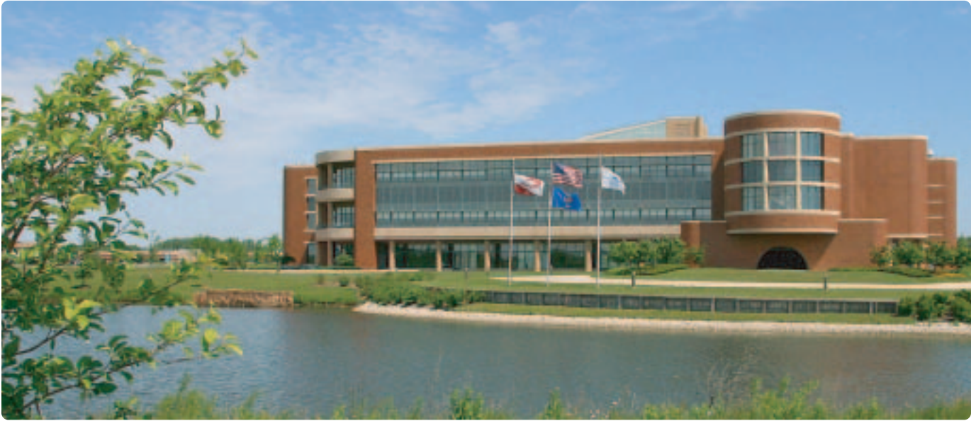
Sophisticated automation is used to measure and control the interior environment in Johnson Diversity's new distribution center in Racine.
